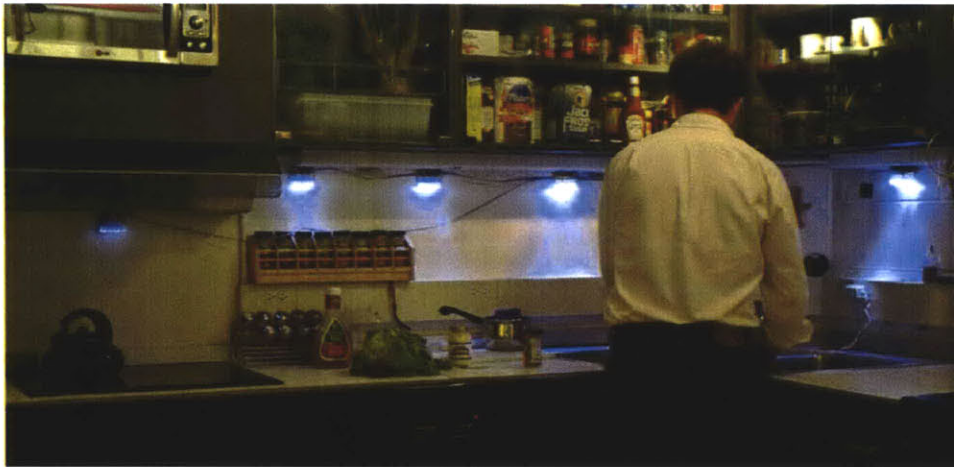
Figure 4-16. Task lights fade in when people perform tasks and fade out when people leave.
